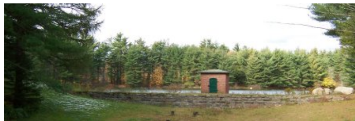
Bristol Water Department Reservoir in the Town of Plymouth.
