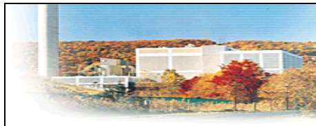
Bristol's "Trash to Energy" Facility owned and operated by Covanta Energy Corp.
