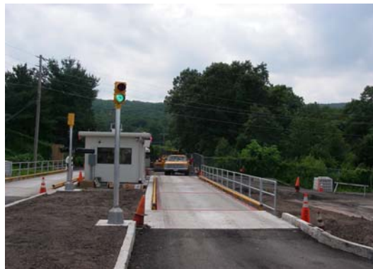
Transfer Station Construction
