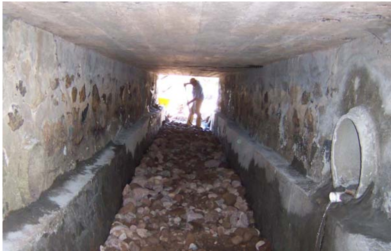
Drainage work on Matthews Street culvert
