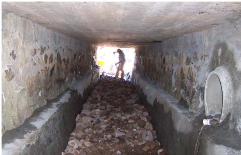
Drainage work on Matthews Street culvert
