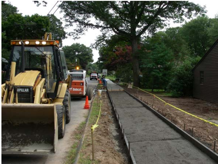
Installation of Sidewalk on Ivy Drive
