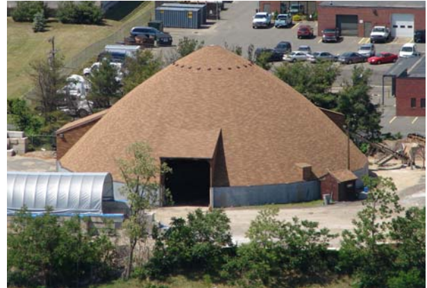
Salt Dome At The City Yard
