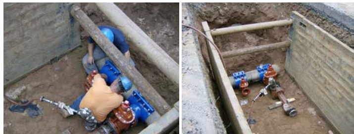
New Service Connection Installation at Business Park Drive.
