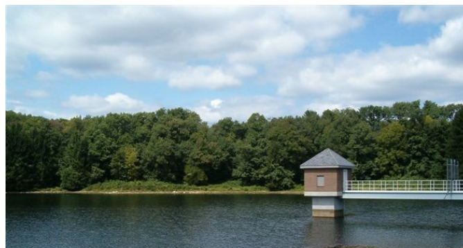
Bristol Water Department Reservoir in the City of Bristol.
