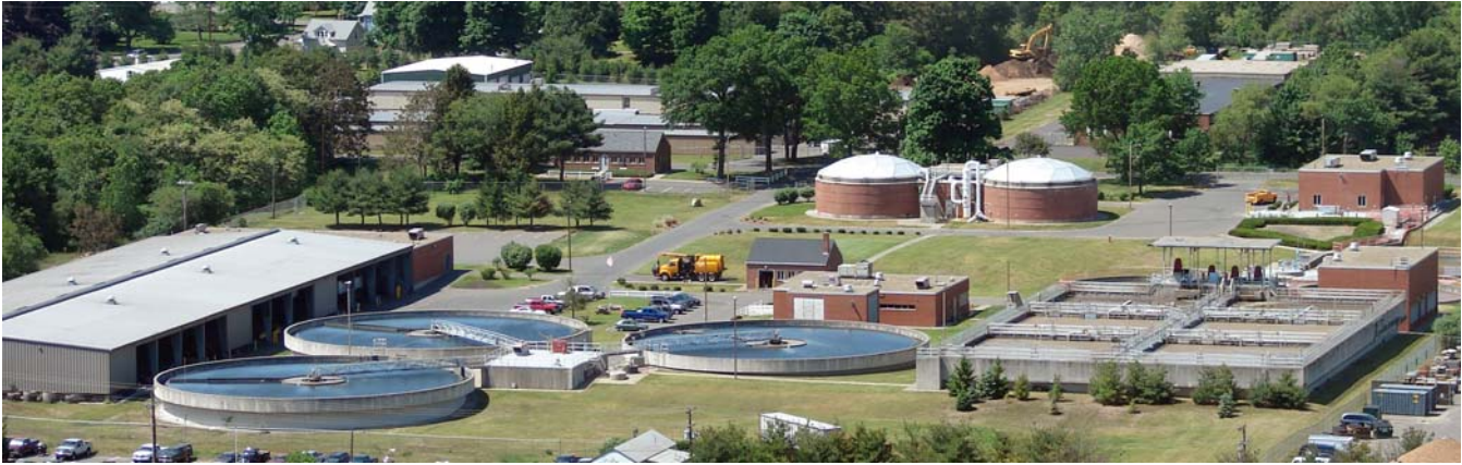
Water Pollution Control Facility
