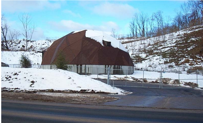
Sand/salt storage dome located on James P. Casey Road.
