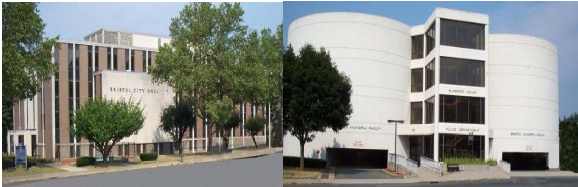
As noted above: City Hall and Police/Court Building
