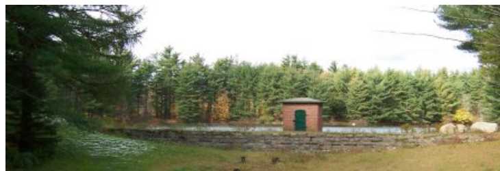
Bristol Water Department Reservoir in the Town of Plymouth.
