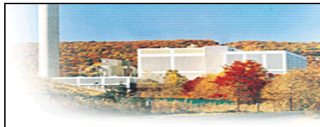
Bristol's "Trash to Energy" Facility owned and operated by Covanta Energy Corp.
